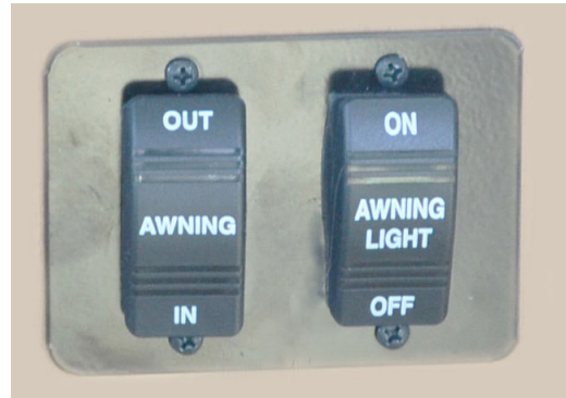
Power Awning Switch and Awning Light Switch (Located near sliding entrance door) -Typical View
