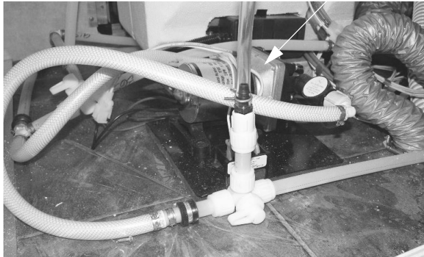
Water Pump (Located at hinged access panel in bed board)) -Model 24V shown
